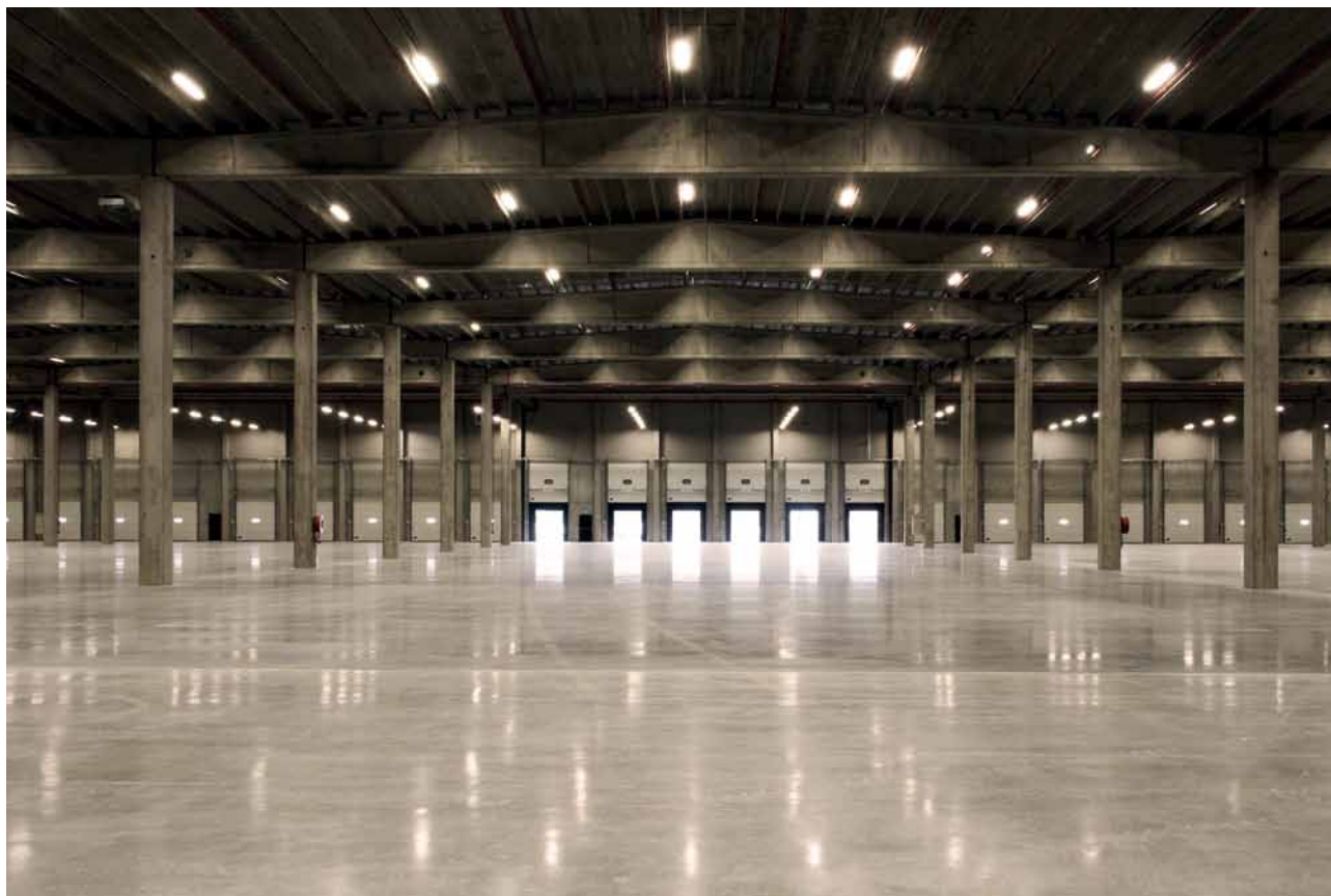
CANAL LOGISTICS - BRUXELLES
