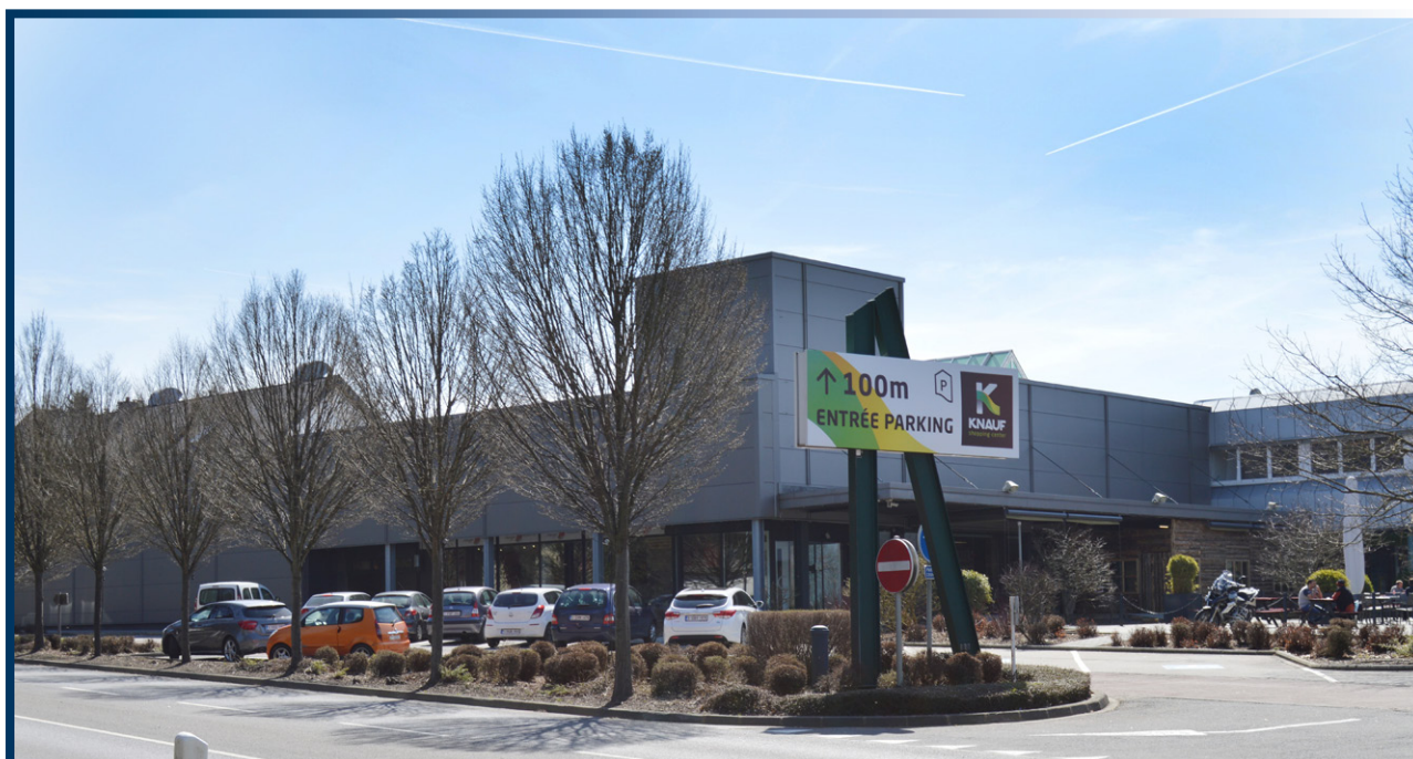
Centre commercial Schmiede, Luxembourg
