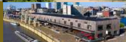
Hangar 26-27 Antwerp (BE) Iconic building Eilandje district € 23 m
