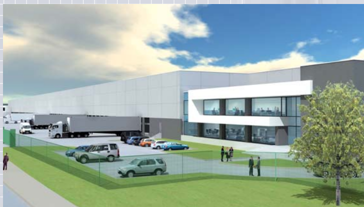
Canal Logistics, Bruxelles
