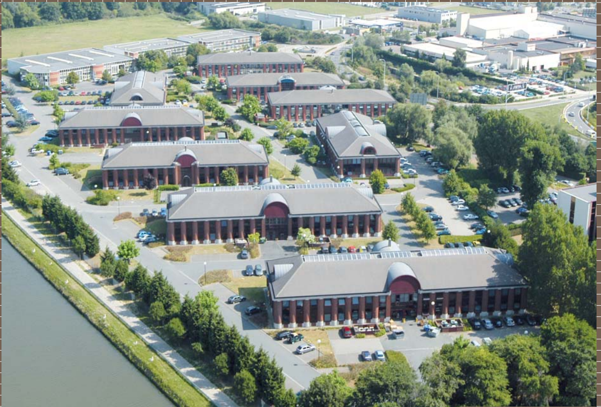
Riverside Business Park, Bruxelles
