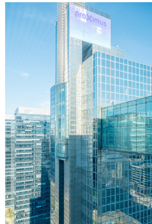
Proximus Towers - Brussels
